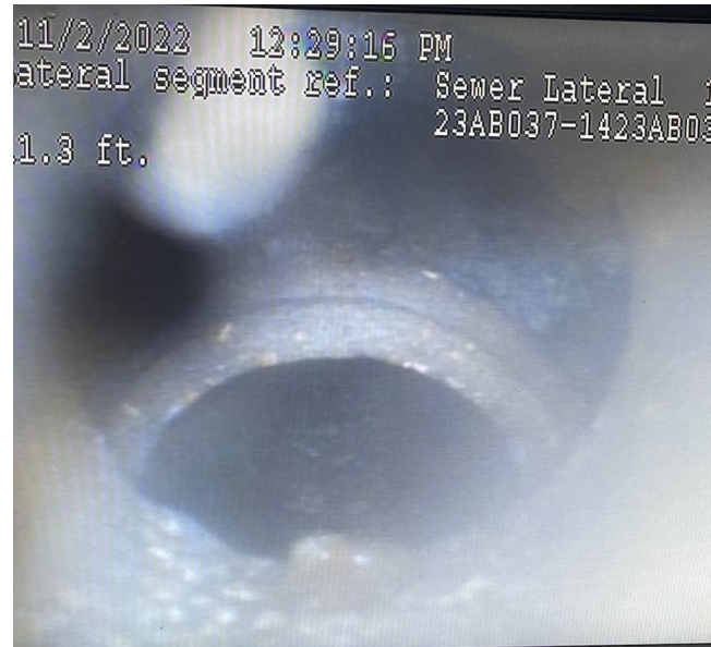
Dropped Pipe Joint
