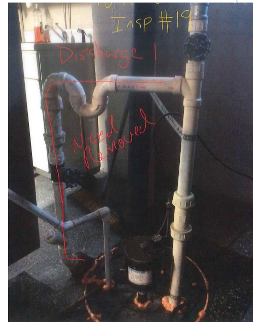
Sump Pump Connected to Sanitary Sewer
