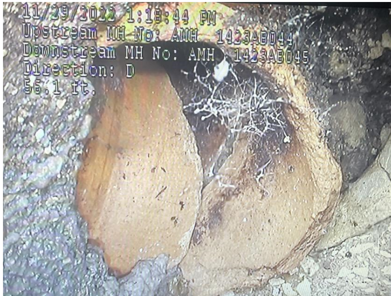
Broken Tap Connection
